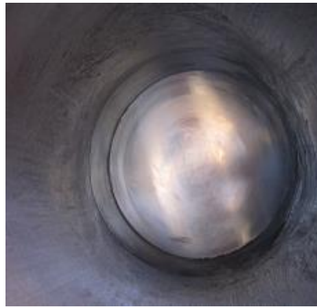
After repair, it is ok!
