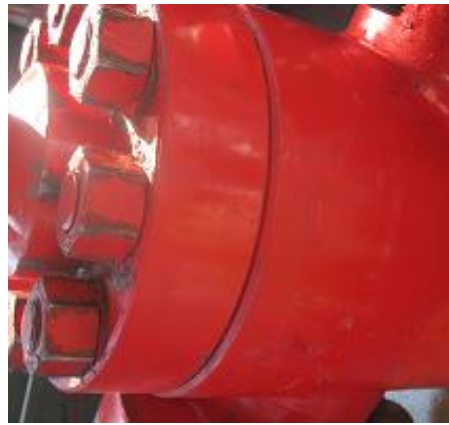
After repair, it is ok!
