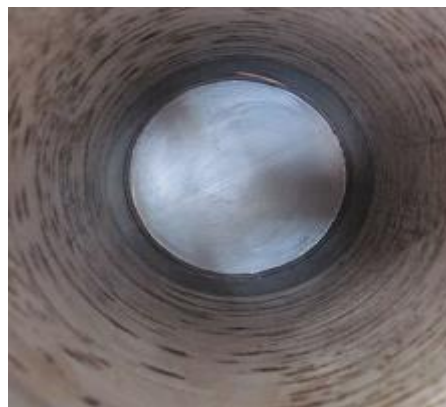
After repair, it is ok!
