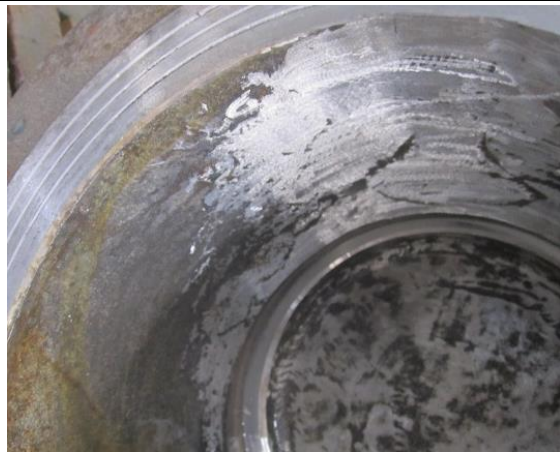
After repairing, it is ok!
