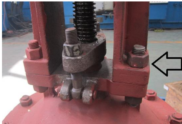
After replacing new one, it is ok!
